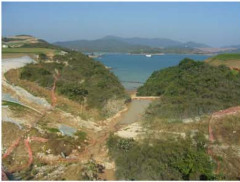
Stream A and the temp bridge area to be restored
