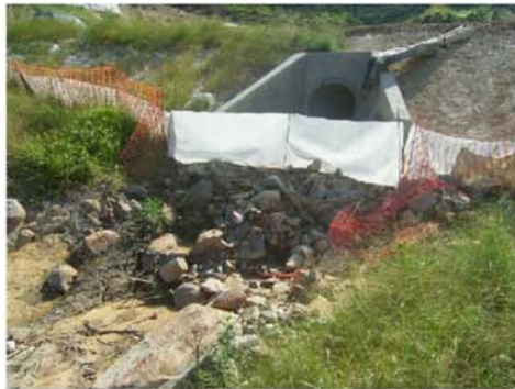
New drain near Stream B2
