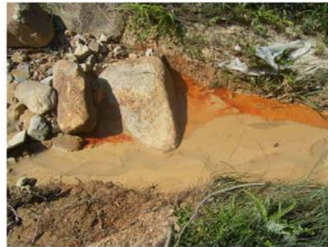
Sedimentation near the new drain
