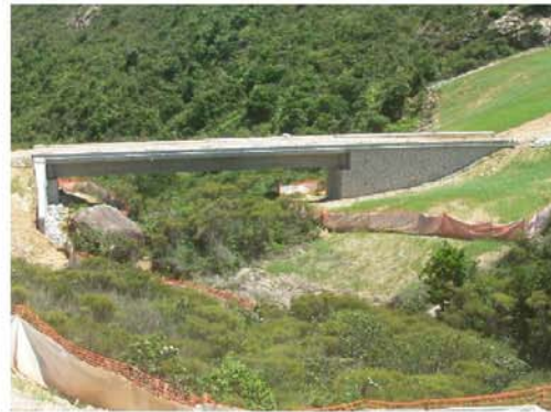
Permanent Bridge in Stream C
