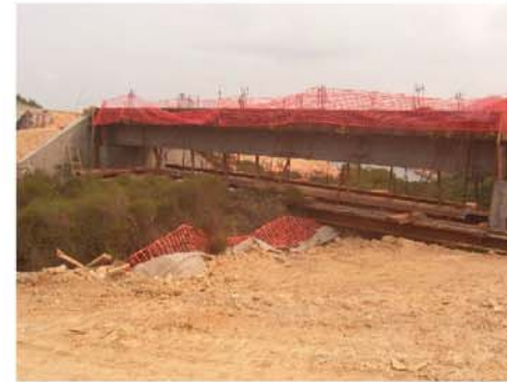
Permanent Bridge in Stream C
